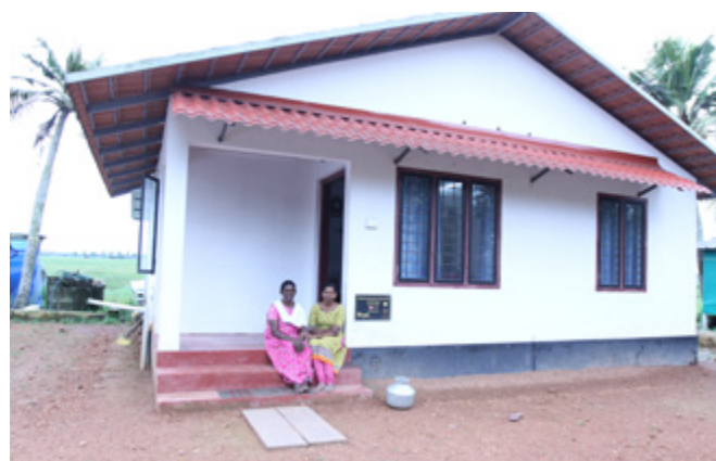
Rebuilding of homes post the Kerala floods
